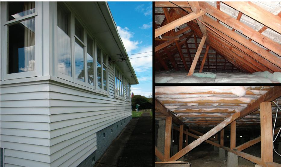
**Figure 4.** North-west facades , hipped roof cavity (timber rafters with concrete tiles and polyester insulation) and basement cavity (jack studs, sleepers and bracing struts on concrete blocks supporting floor joists with polyester insulation in-between) of the pilot project house in 2012.
