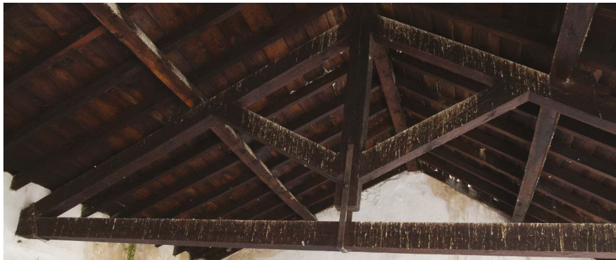
Figure 6. Gallery; detail of an open-node truss.
