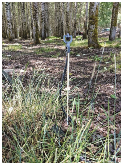
Figure 5. One of the 20,000 sprinkler heads used to irrigate the Chehalis Poplar Tree Plantation with reuse water.
