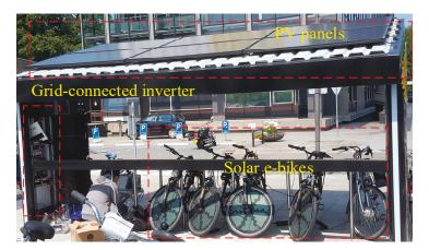
**Figure 1.** The PV (photovoltaic)charging station with 6 PV modules (top), a grid-connected inverter (at left column), and 4 solar e-bikes that are being charged.
