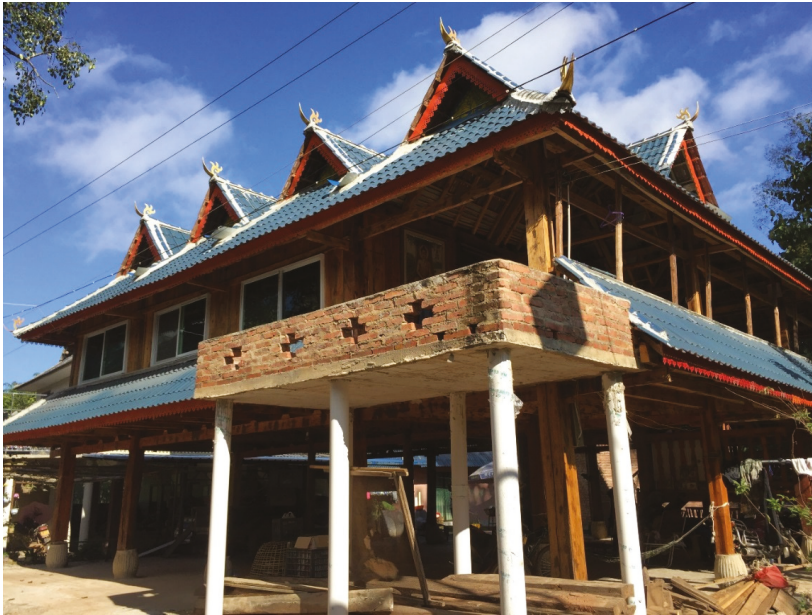
Figure 5. Hybrid style of dwelling (under construction).
