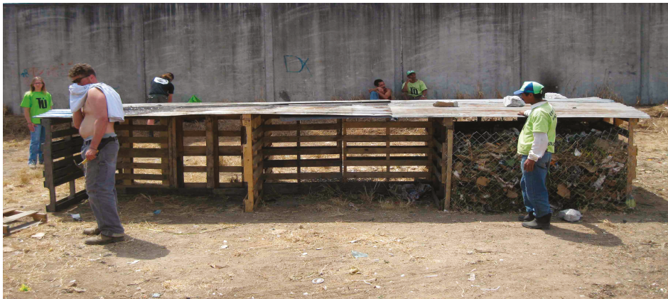
Figure A10. An image of the three-cell hybrid compost bin system adapted for the Guatemala test project.
