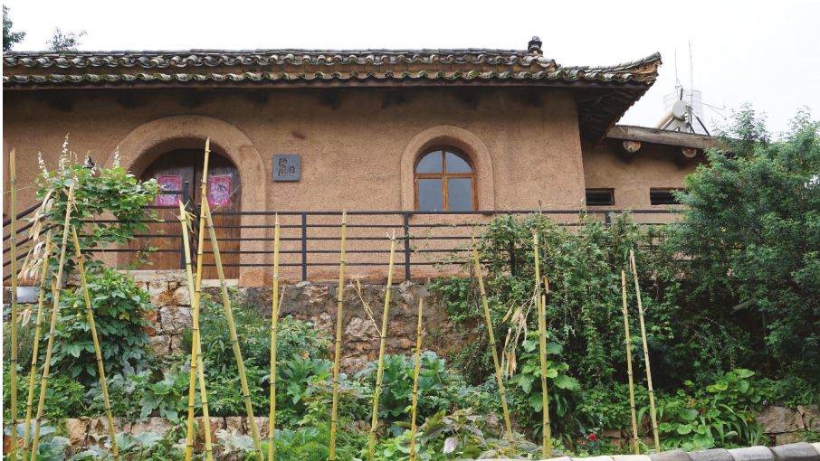
Figure 6. Damoyu—renovated mud and straw brick/adobe building.
