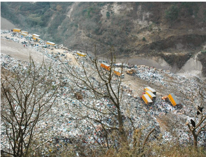
Figure A5. The landfill is expansive, very dangerous, prone to landslides, and emits methane gas from decomposing waste material.
