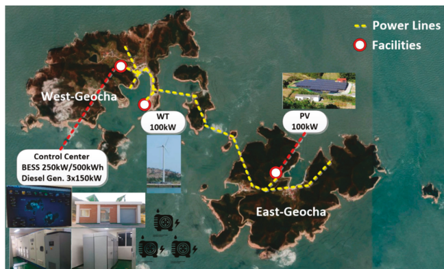
Figure 1. Isolated microgrid on Geocha Island, South Korea.
