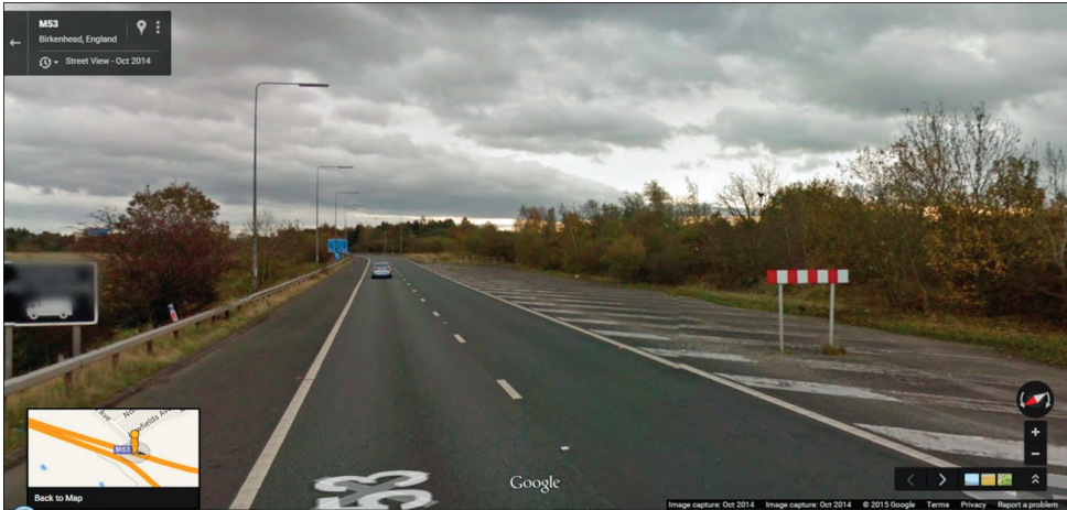
Figure 13. View approaching the island on the southbound carriageway (Map data: © Google [2014]).
