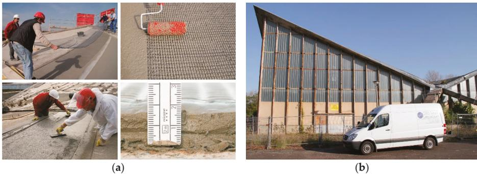
**Figure 6.** Textile reinforced concrete (TRC) retrofitting of hyper shells; (a) application of TRC strengthening at a hyper shell in Schweinfurt (photos: Ulrich van Stipriaan and Silvio Weiland, reproduced with permission from [59], Ernst & Sohn, 2015), (b) hyper shell in Magdeburg before restoration (photo: Heiko Wachtel).
