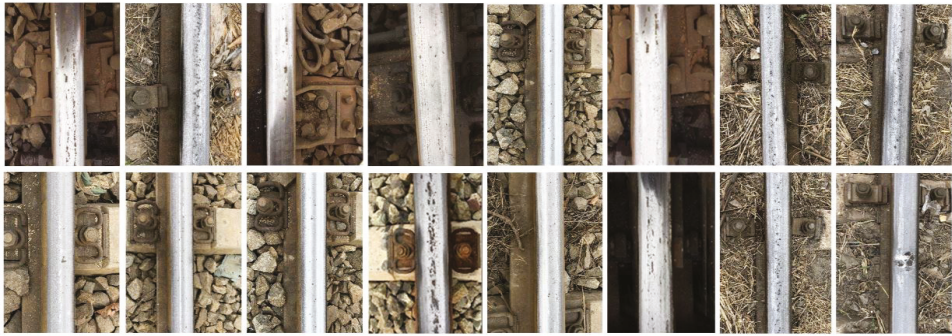
Figure 9. Examples of UAV images containing discrete defects on rail surfaces.
