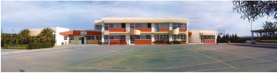
Figure 2. General view of the examined school building.
