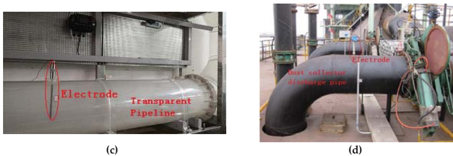
Figure 1. Working principle figure of the electrode and its application: (a) Schematic figure; (b) in the iron mining company; (c) in the laboratory; and (d) in the steel mill company figure.
