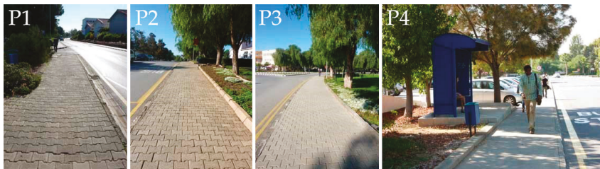
Figure 3. Quality of payments, shading elements and width of pedestrian paths: P1 Quality of payments along pedestrian paths within EMU Campus; P2–P3 Trees being the only elements providing shade for pedestrians along the sidewalks; P4 —Insufficient width of pedestrian paths along the main axis (Source: Authors).
