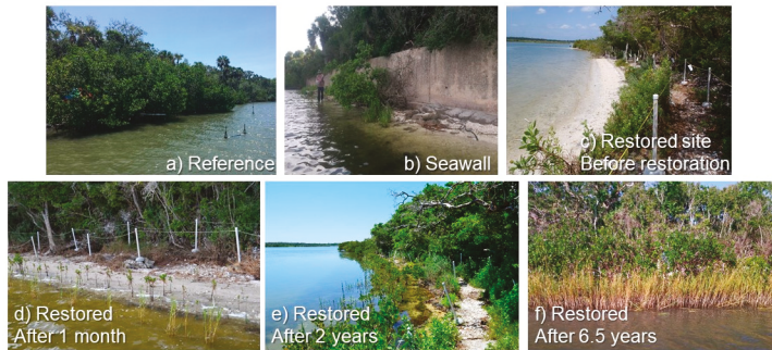
Figure 2. Study sites: (a) Reference shoreline site with mature mangrove vegetation; (b) Seawall shoreline site at the time of hydrodynamic data observation, four years after hybrid shoreline restoration; (c) Restored shoreline site before restoration; (d) Restored shoreline site one month after restoration; (e) Two years after restoration; and (f) at the time of hydrodynamic data observation, 6.5 years after restoration.
