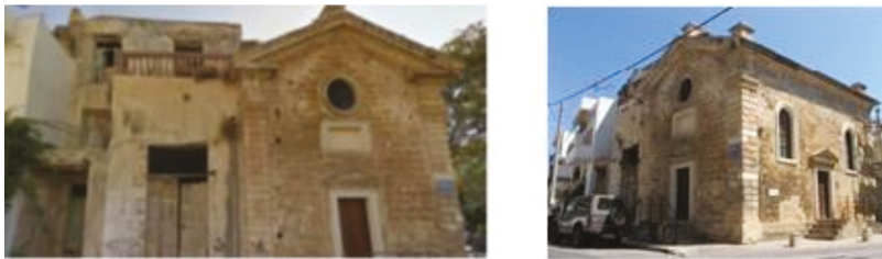
Figure 2. Front side of the temple showing the northern (left) and the southern (right) part.
