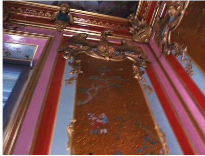
Figure 11. Example of the details under a high ceiling.
