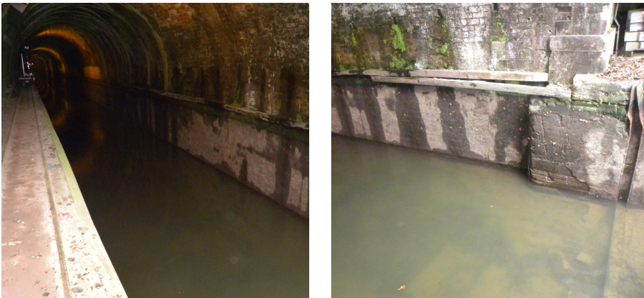
Figure 3. Entrance of Arzviller's tunnel during its emptying in 2009.
