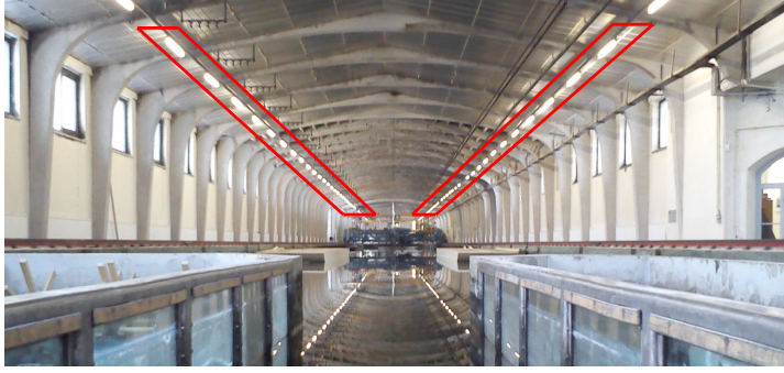
Figure 8. Two arrays of lamps are marked with red bounding boxes. The end points of the single lamps served as the control information.
