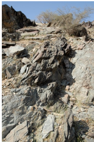
Figure 6. Highly fractured pelitic rocks consisting of schists and meta-shales along the Wadi Qidayd perimeter.
