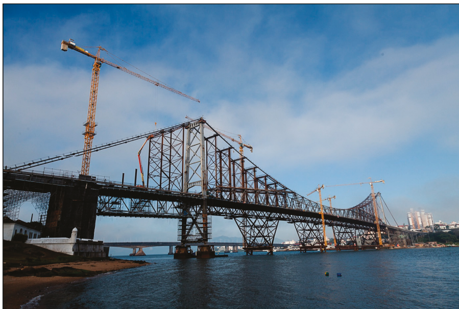
Figure 9. A view of the Hercílio Luz Bridge, reproduced with permission from Eduardo Trauer (photo taken in February 2018).
