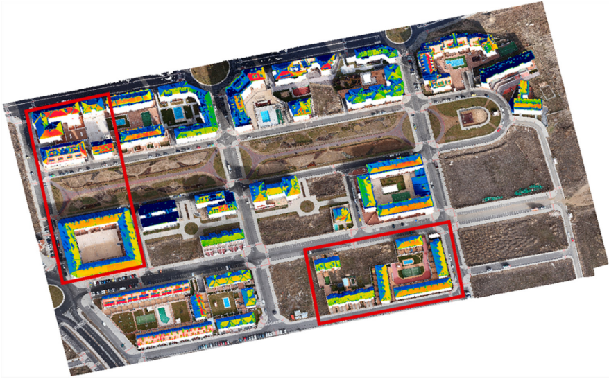
Figure 7. Hybrid 3D point cloud generated from images captured with the RGB camera integrating thermographic texture mapped over the roofs. Areas shown in detail in consecutive figures are remarked in red.
