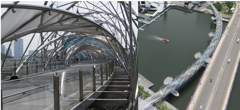
Figure 3. The Helix Bridge is a pedestrian bridge in the Marina Bay area in Singapore. Its generative design has been optimized numerically. Furthermore, the bridge was fully modeled in order to visualize its form and geometrical compatibility, as well as to visualize the pedestrian experience on the bridge.
