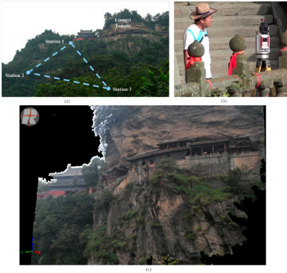
Figure 5. Long-distance laser scanner was used to acquire 3D data of the cliff terrain, and the scanning stations were located throughout the whole building (a); (b) scanning work scene on the platform; (c) 3D point cloud data with color information.
