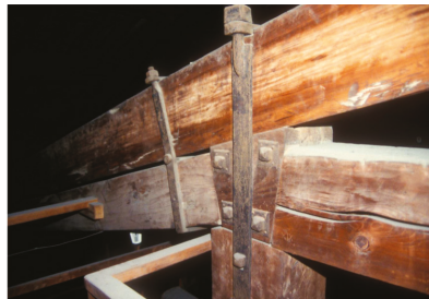
Figure 9. Salone dei Cinquecento, Palazzo Vecchio, Florence, Italy: Detail of timber roof structure and iron fasteners (the iron reinforcement is part of the original structure from 17th century).
