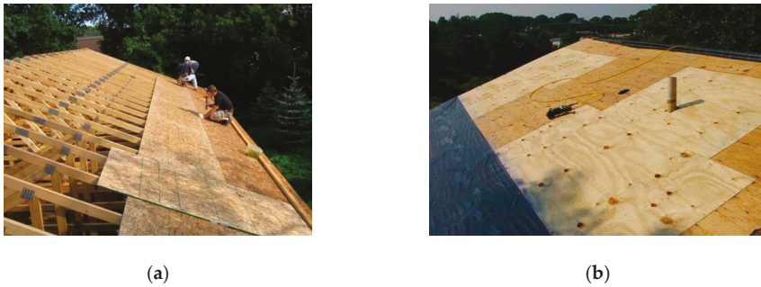
Figure 30. Examples of use of wooden boards.
