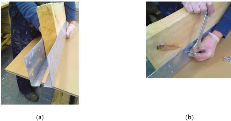
Figure 11. Re-construction of joist ends with stainless steel L-shaped profiles (press-bended stainless steel sheets) [43].
