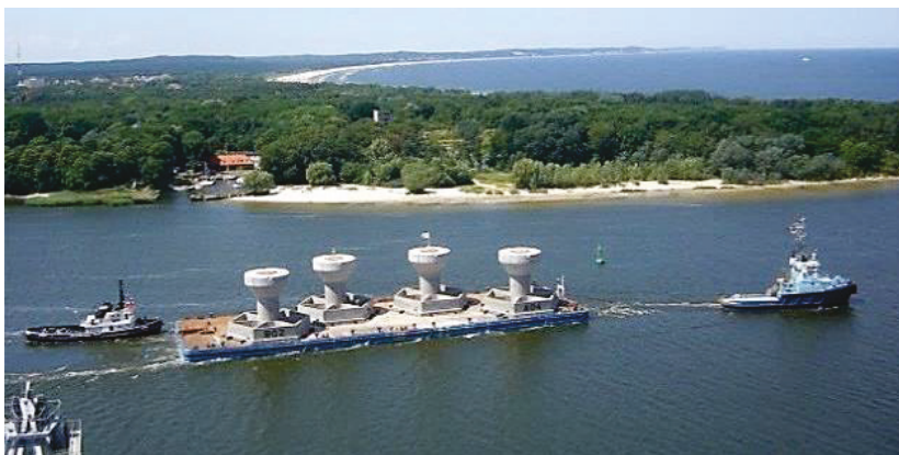
Figure 3. Lillgrund offshore wind farm foundations reproduced from [21], with permission from Tech-Marine, 2019.
