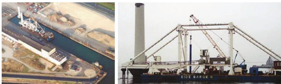
Figure 1. Middelgrunden offshore wind farm foundations, reproduced from [20], with permission from Elsevier, 2019.
