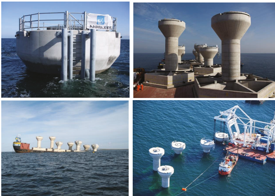
Figure 4. Sprogø offshore wind farm foundations [22], with permission from Aarsleff, 2019.
