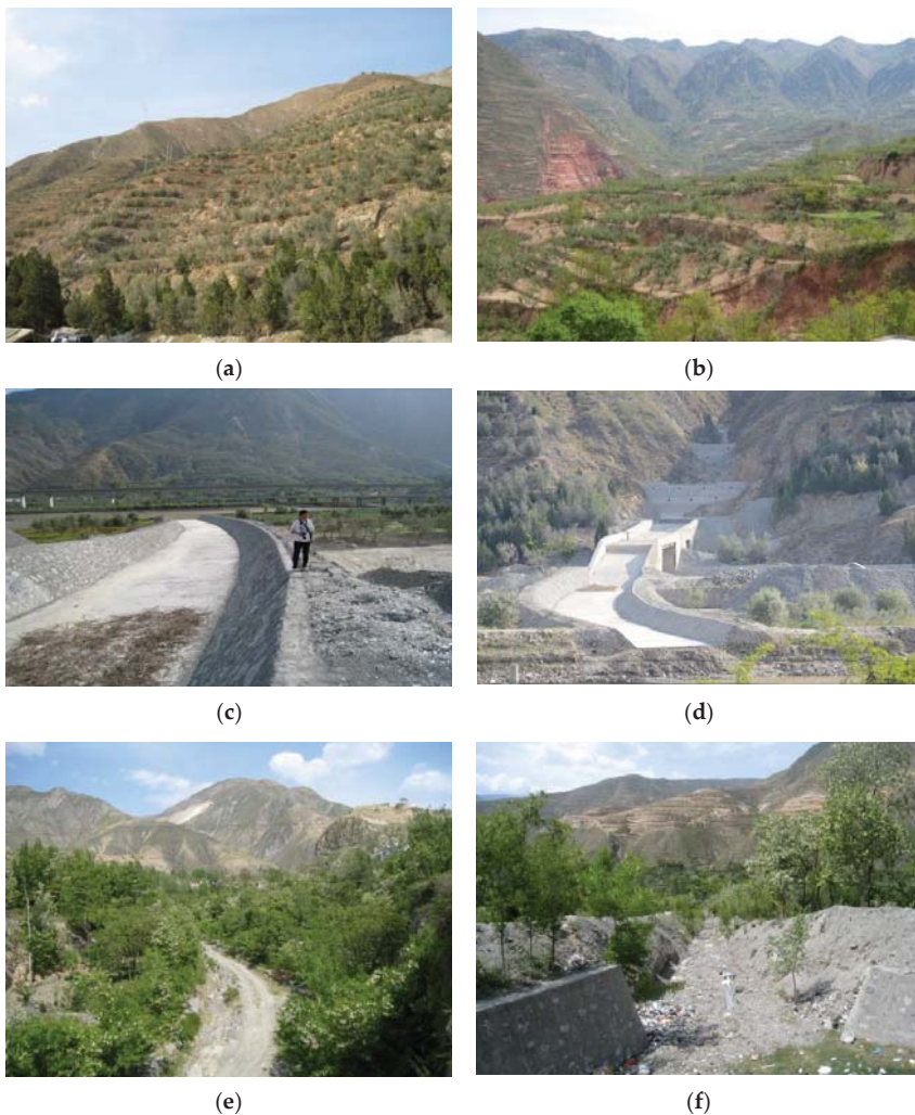
Figure 7. Various measures for ecological preservation: (a,b) Slope ecological protection measures; (c,d) drainage groove with check dam; (e,f) ecological engineering protection in gully.
