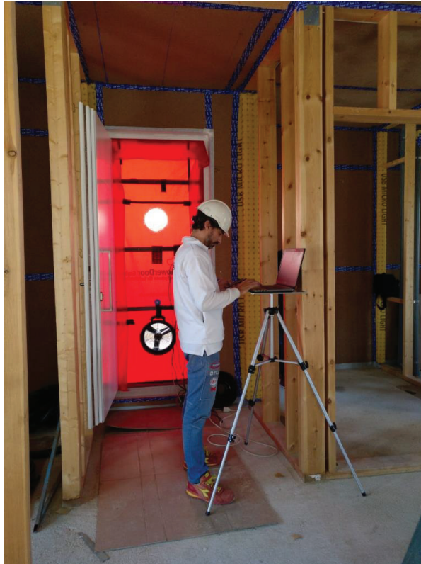
Figure 7. Image during the Blower Door test; 3 October 2018.
