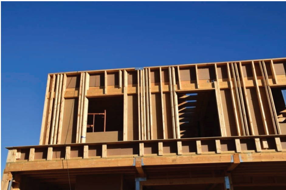
Figure 3. View of the southeast façade. Construction of enclosures and floors.
