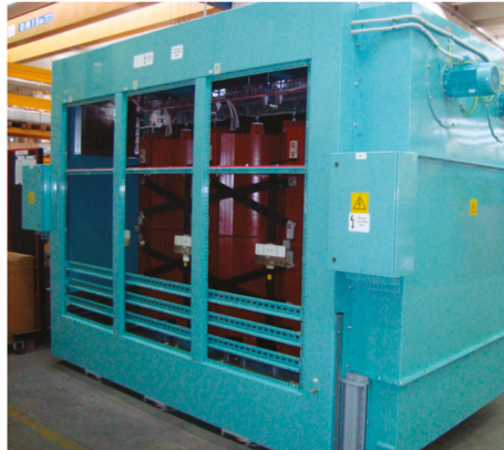
Figure 4. Phase shifting transformer installed on large-scale electric propulsion system.
