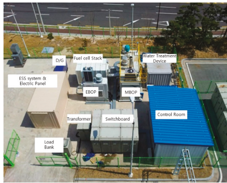
Figure 3. Actual placement of the test bed.
