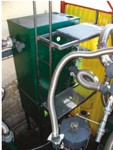
Figure 2. Sleeve filter for trapping solid particles (SP).
