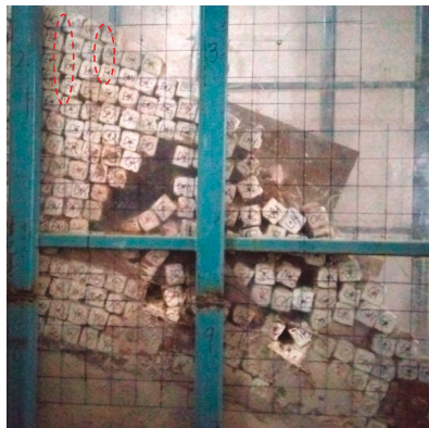
(a) Deformation after mining ore body #4
