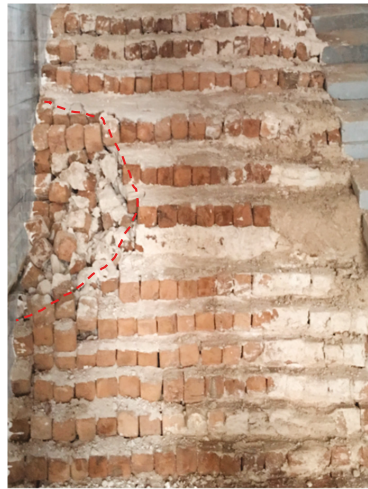
Figure 13. Front view of the model slope after four stages of mining. Subsidence pit was formed above the mining area.
