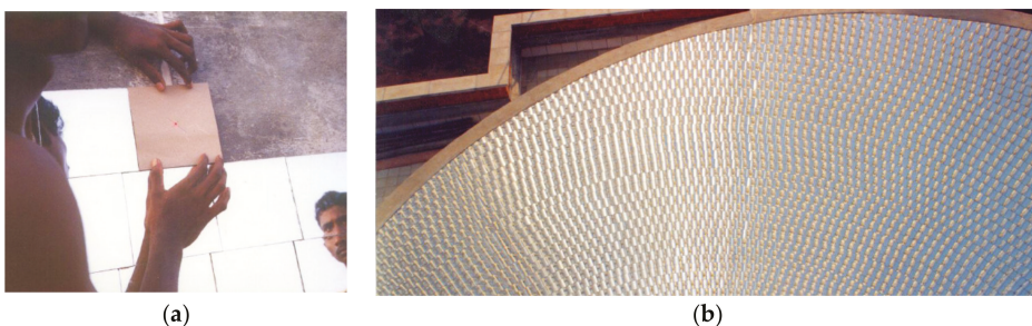
Figure 6. Small facets glued to the spherical concrete bowl in Auroville, India [15]: (a) Gluing and canting process; (b) Mirrors seen from the center of the sphere.
