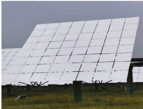
Figure 4. Surface shape of heliostat in the Yanqing CSP plant.
