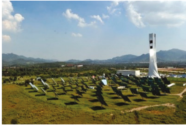
Figure 1. A perspective view of the heliostat field in the Yanqing concentrated solar power (CSP) plant.
