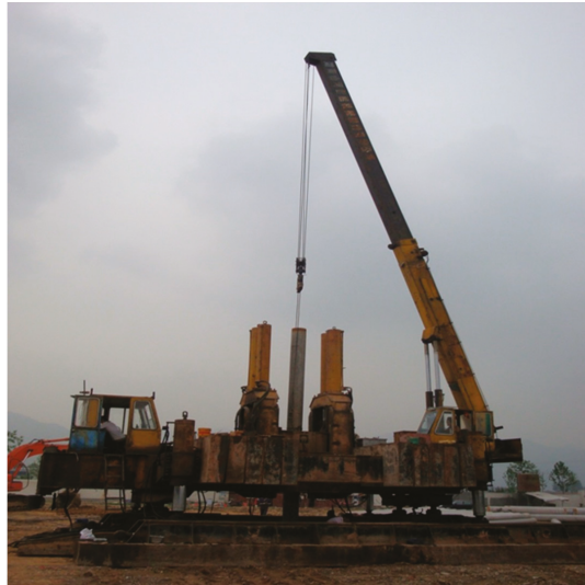
Figure 4. Jacking machine used in the test.
