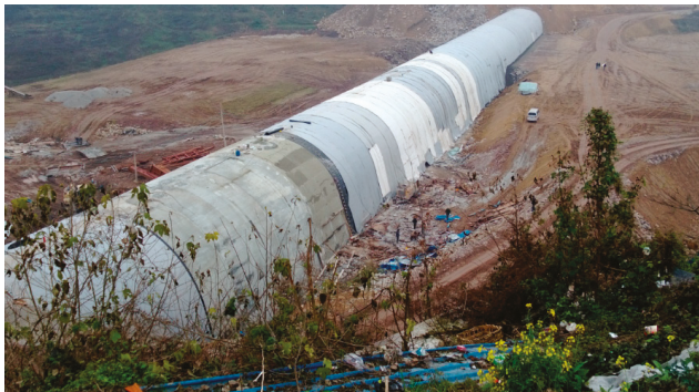
Figure 5. Open-cut tunnel in the backfill process.
