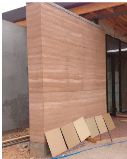
Figure 1. Wall made from compacted earth. The compacted layers of mixed soil are shown.
