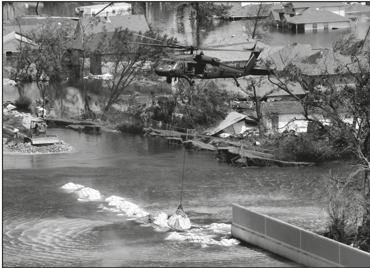
Figure 10. Black hawk dumping sandbags to close the 17th Street Canal levee breach [29].
