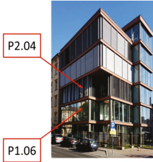
Figure 1. Location of test room P2.04 (with external venetian blinds) and P1.06 (with no venetian blinds).
