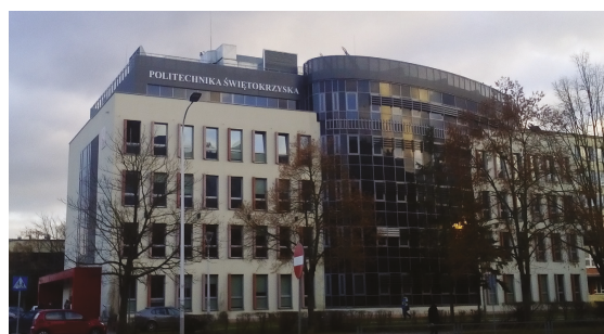
Figure 1. “Energis” building of Kielce University of Technology (Western façade).
