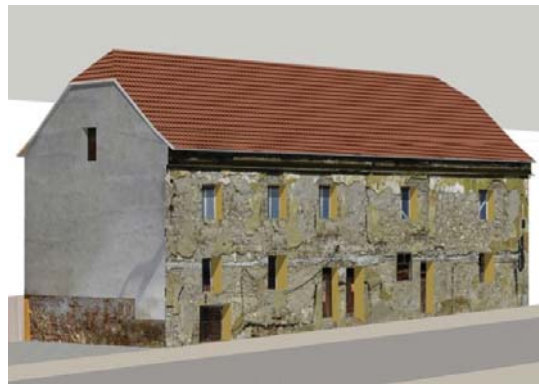
Figure 7. Real view of Strejc’s Church in Židlochovice (CR).
