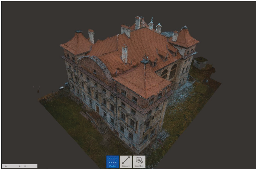
Figure 4. Point cloud converted with Autodesk ReCap software.
