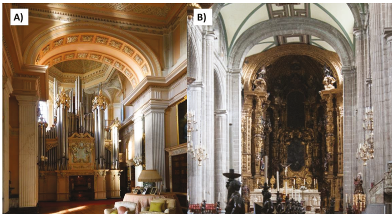
Figure 6. (A) Basket-handle arch of one of the galleries of the Blenheim Palace (UK). (B) Basket-handle arch of the central nave of the Metropolitan Cathedral of Mexico City.
