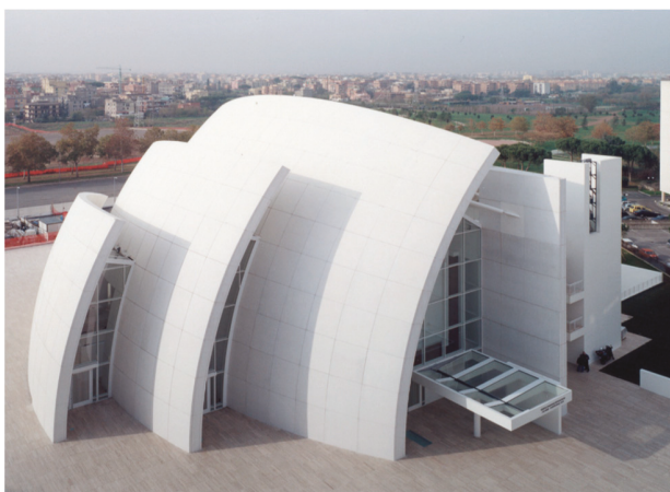
Figure 47. Dives in Misericordia Church, Rome, constructed of TiO 2 self-cleaning and depolluting TX Active cement (inaugurated in 2003). Reproduced from https://es.i-nova.net/content?articleId=96804 or https://www.archdaily.com/20105/church-of-2000-richard-meier .
