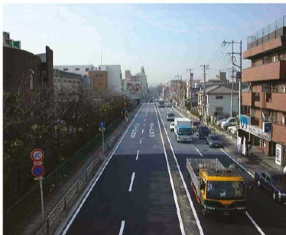
Figure 29. Usage of TiO 2 -based photocatalytic material on roadway surfaces to convert nitrogen oxides NO x to nitrate: finished roadway with the coated surface showing a lighter color—photo was courtesy of Fujita Road Construction Co., Ltd. to the authors of Ref. [117]. Reproduced with permission from Fujishima et al. [117]. Copyright 2008 by Elsevier B.V. (License No.: 4452671501245).
