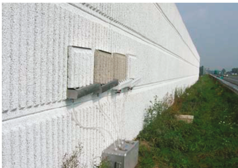
Figure 51. Example of a \text{TiO}_2 -coated concrete noise barrier erected along the A1 and A28 highways in Terschuur and Putten, the Netherlands. Reproduced from Ref. [152].
