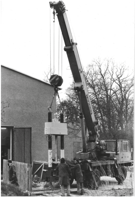
Figure 3. Assembling the triaxial press.
