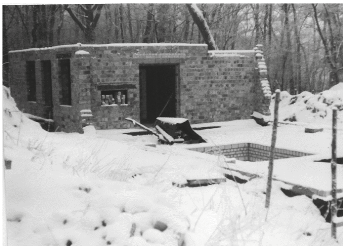
Figure 2. Construction site of the first high pressure hall with a pit for the triaxial press (6 January 1971).
