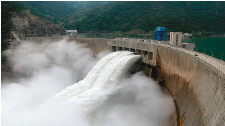
Figure 1. Simultaneous discharge of the surface and the deep hole of the Ertan hydropower station in 2010.
