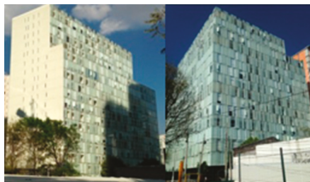
Figure 5. Photographs of the building under study.
