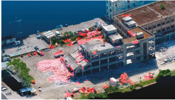
Figure 4. Point cloud representation of an INACHUS pilot structure in Lyon, France, calculated from optical imagery acquired with a low-cost commercial drone (Phantom 4, DJI), showing damage detected through machine learning (red).
