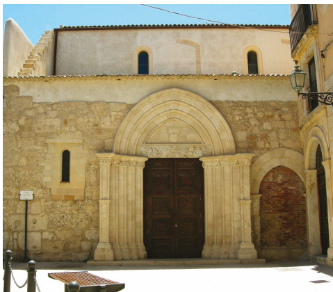
(a) Northern façade
