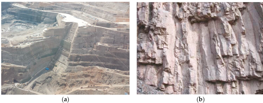
Figure 11. Site conditions of the Baihetan Hydropower Station: (a) construction site, and (b) typical columnar jointed basalt.
