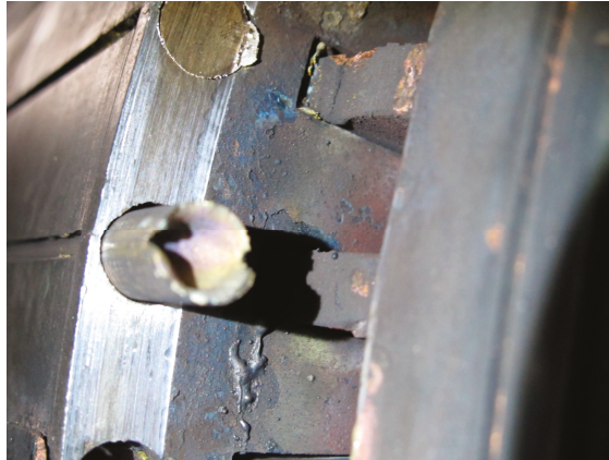
Figure 1. Damaged rotor cage, view after cutting off the end ring of the starting cage—visible melting of the starting cage bar.
