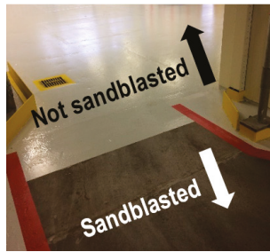
Figure 5. An example of a sandblasted and not sandblasted pallet mover transportation route.
