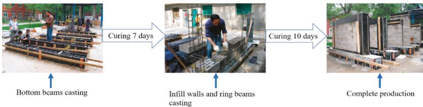
Figure 4. Process of the construction of masonry wall specimens.
