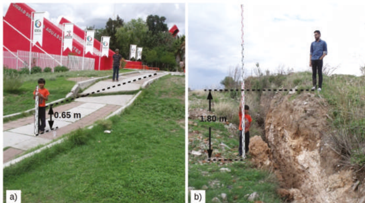
Figure 1. Surface faults due to differential subsidence in Aguascalientes. (a) Surface fault affecting man-made structures; (b) Surface faulting has developed escarpments up to 1.80 m high. The location of the subsidence-related surface faults is shown in Figure 2b.
