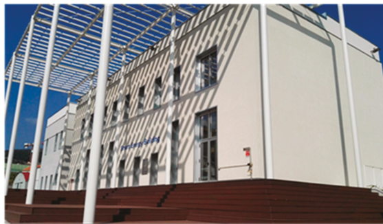
Figure 4. The Smart Energy Building.
