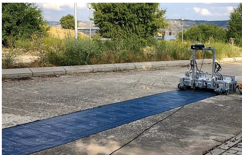
Figure 22. Asphalt roll installation.
