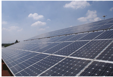
Figure 6. Physical system for the Mexico City site (MCS).
