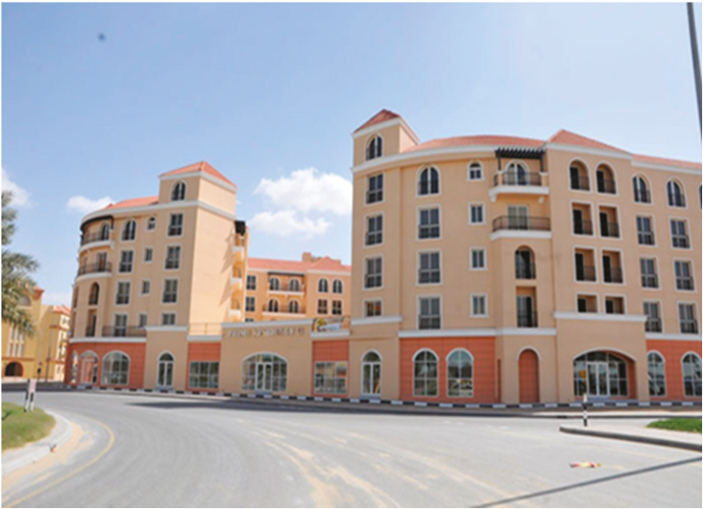
Figure 3. Prime Residency II (PR II), International City, Dubai, UAE.
