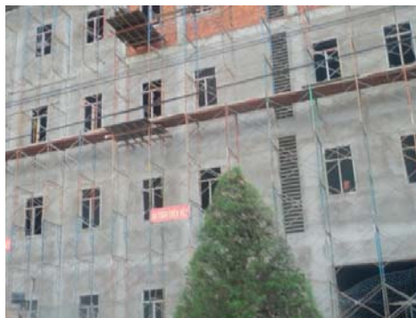
Figure 3. An industrial building under construction in Can Tho City.
