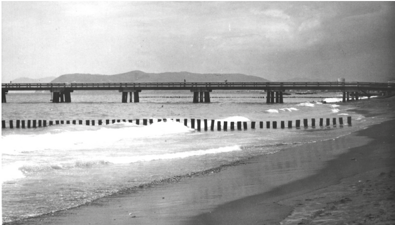
Figure 10. Marina di Massa: permeable groins in a picture taken in 1968 (the pier in the background).
