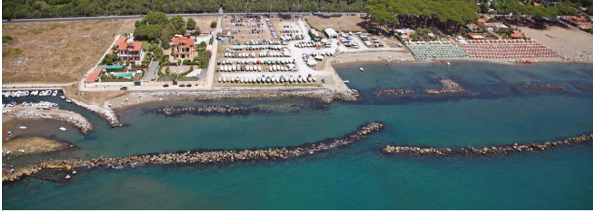
Figure 9. Marina di Carrara: area downdrift of the harbour with different defence structures (Photo Provincia di Livorno).
