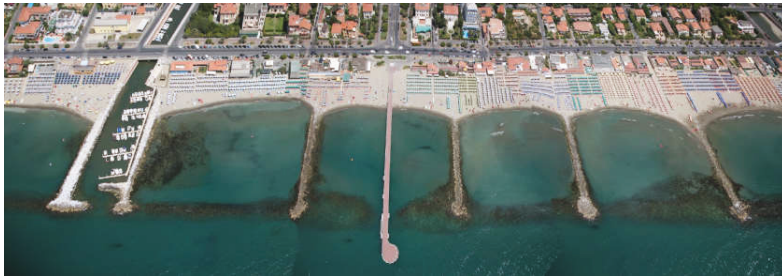
Figure 11. Groins with tips connected by submerged breakwaters. On the left the Brugiano R. with jetties; on the centre the Marina di Massa pier (Photo Provincia di Livorno). Summer shot captures sun umbrella density.
